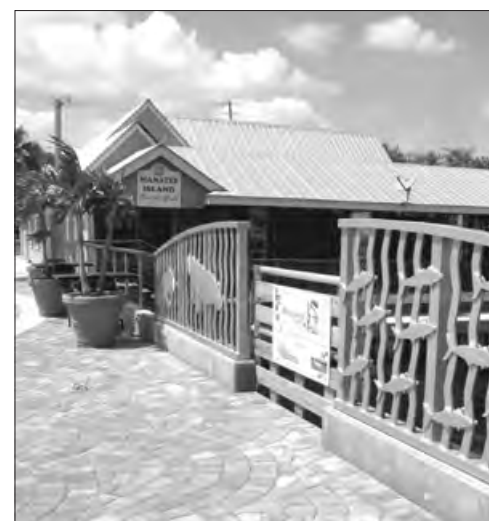
Manatee Island Bar & Grill in Port Salerno will construct a portion of the CRA's Manatee Pocketwalk adjacent to its restaurant with private funds.
