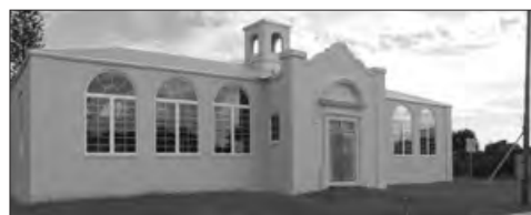
Apollo School in Hobe Sound now has new windows installed, new stucco on its walls, and new electrical wiring inside. An Open House on Oct. 13 will be the first opportunity for the public to view the restored building.
