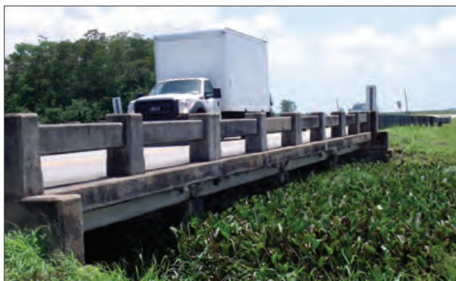
Bridge Road will be closed between I-95 and Pratt Whitney Road intersections as soon as the 2013 school year ends in order to replace a weight-restricted bridge that county engineers have deemed obsolete.
