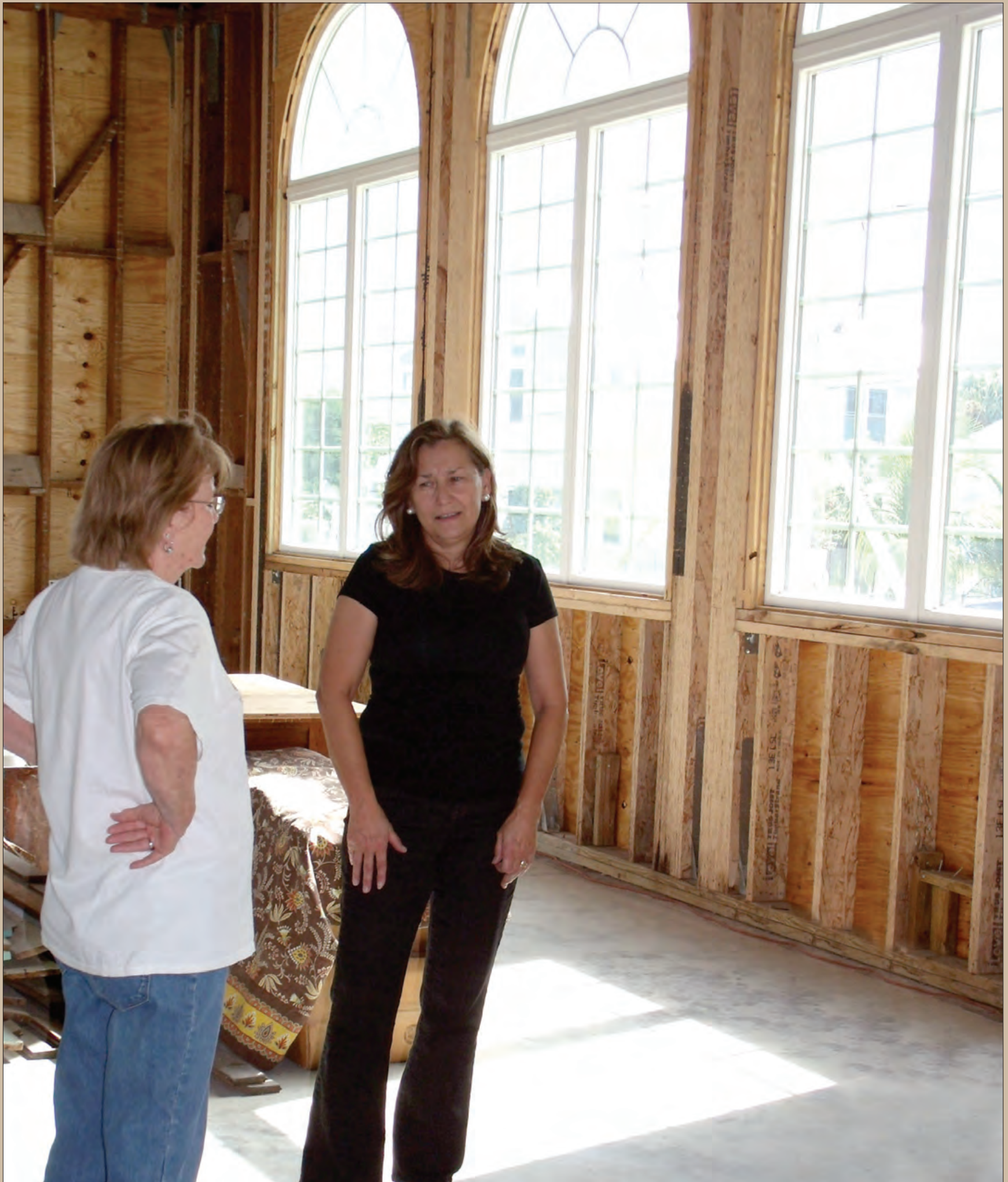
THE APOLLO SCHOOL -- The public's first look at the inside of the partially restored Apollo School in Hobe Sound came early in October as part of the Martin County Historic Preservation Month celebration. Much work, including new windows, has been completed, but much more remains to be done, according to Kathy Spurgeon, head of the Apollo School Foundation. Volunteers Miriam Holt, left, and Mary Cox spent the day greeting guests who stopped by to get a glimpse of the past.
