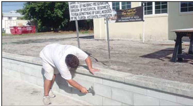
Historic preservation makes progress at the Apollo School in Hobe Sound as Marc Collette of Concrete Transformations puts finishing touches on the renovated school's new retaining wall to give it a more aged look.
