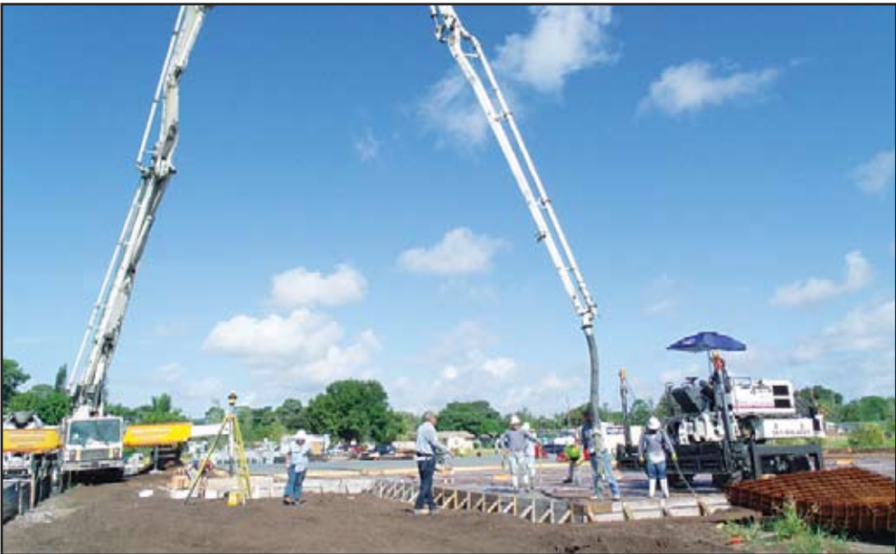
Cement is being poured and leveled for the new 20,000 sq.ft. Boys & Girls Club at the heart of Carter Park at Indiantown.
