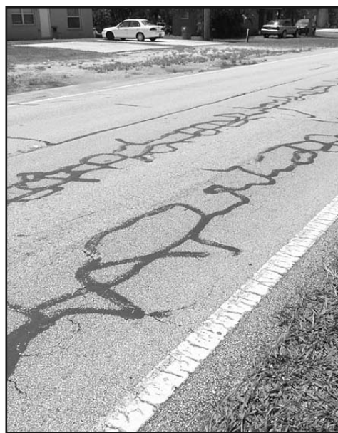
Indian Street wears the crack-sealed dress becoming more common on Martin County roads.
