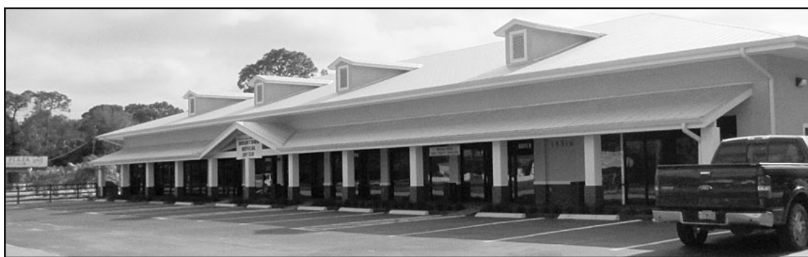
The Indiantown Community Service Center at 15516 SW Osceola Street in Indiantown that will house the new iTown Medical Center.
