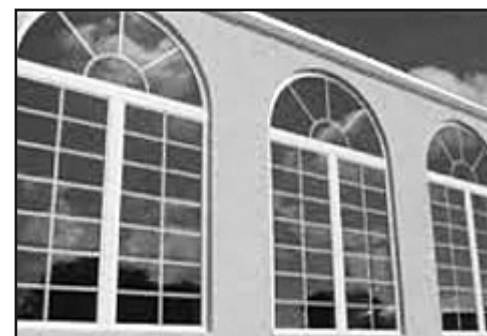
The distinctive windows of the Apollo School are one of the renovations of the historic building in Hobe Sound that will be celebrated with an official ribbon-cutting and community celebration at the school March 29 at 10 a.m. The public is invited to attend.
