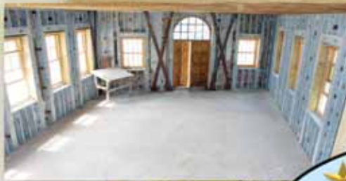
THE INTERIOR OF THE BUILDING remains unfinished, although it has been reinforced. The photo is taken from the top of the stairs looking toward the front door.
