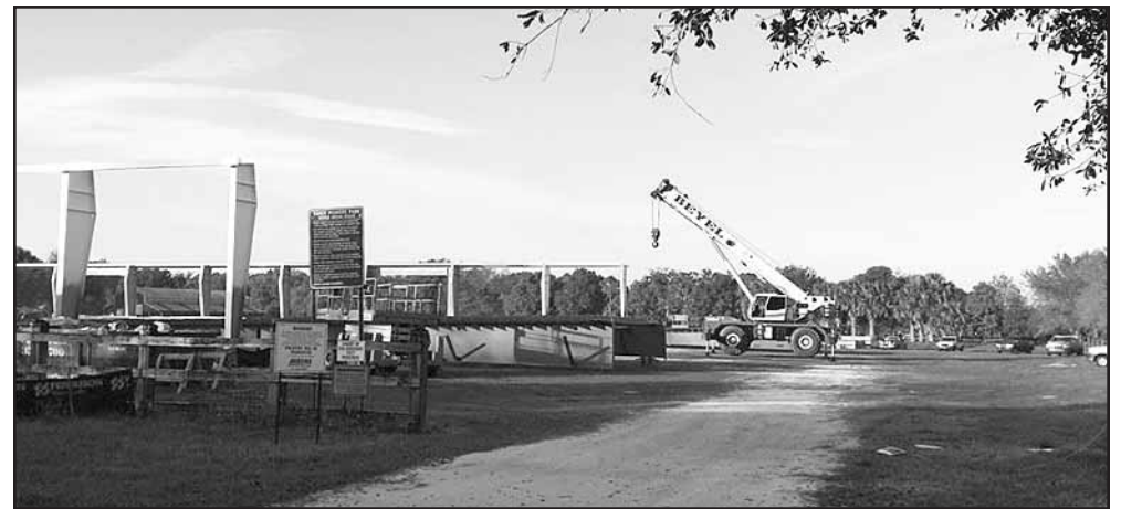
The Timer Powers Park arena roof first began to take shape with the placement of its "legs," huge beams that towered above the landscape.
