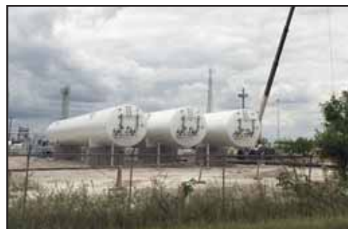
The storage tanks for the liquefied natural gas are in place at the Medley plant, ready to hold the 100,000 gallons of LNG produced daily to fuel FEC trains and to export internationally.
