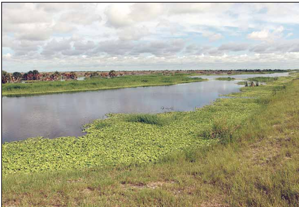
Some of the canals are covered completely with water lettuce and hyacinths, which will need to be removed mechanically to keep the water farm functioning at peak levels.
