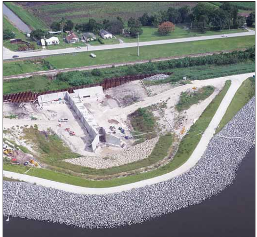
An aerial view of the progress in repairs of the Herbert Hoover Dike around Lake Okeechobee. After repairs are completed, a dam study will be completed that could lead to a re-evaluation of the Lake Okeechobee Regulation Schedule that determines timing and amount of the fresh water discharges from the lake.
