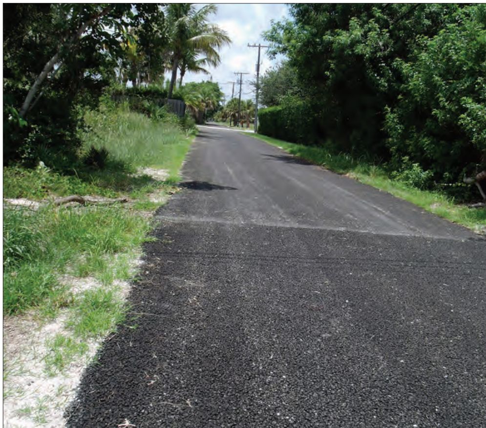
Pervious asphalt now covers Old Post Office Alley in Hobe Sound.
